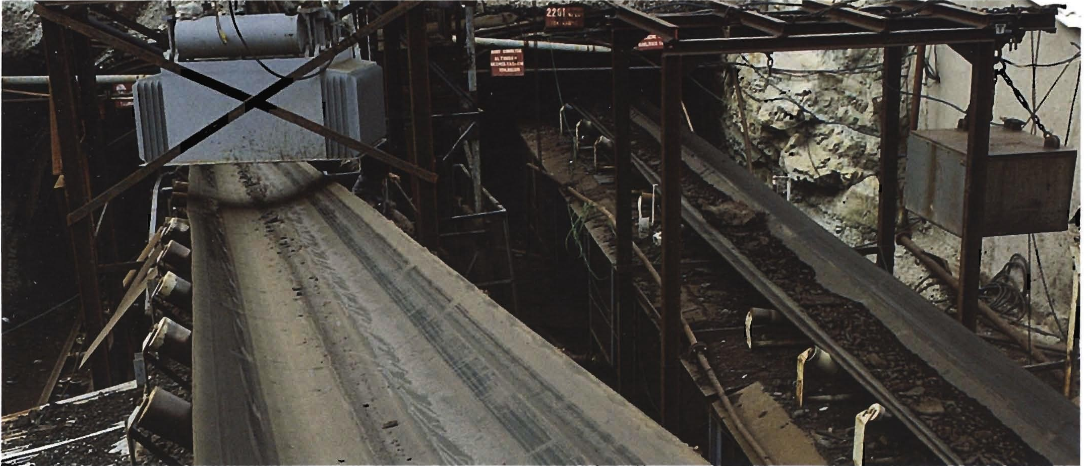
▼ Underground Coal Belt / ST - 1000 / 1200 mm
