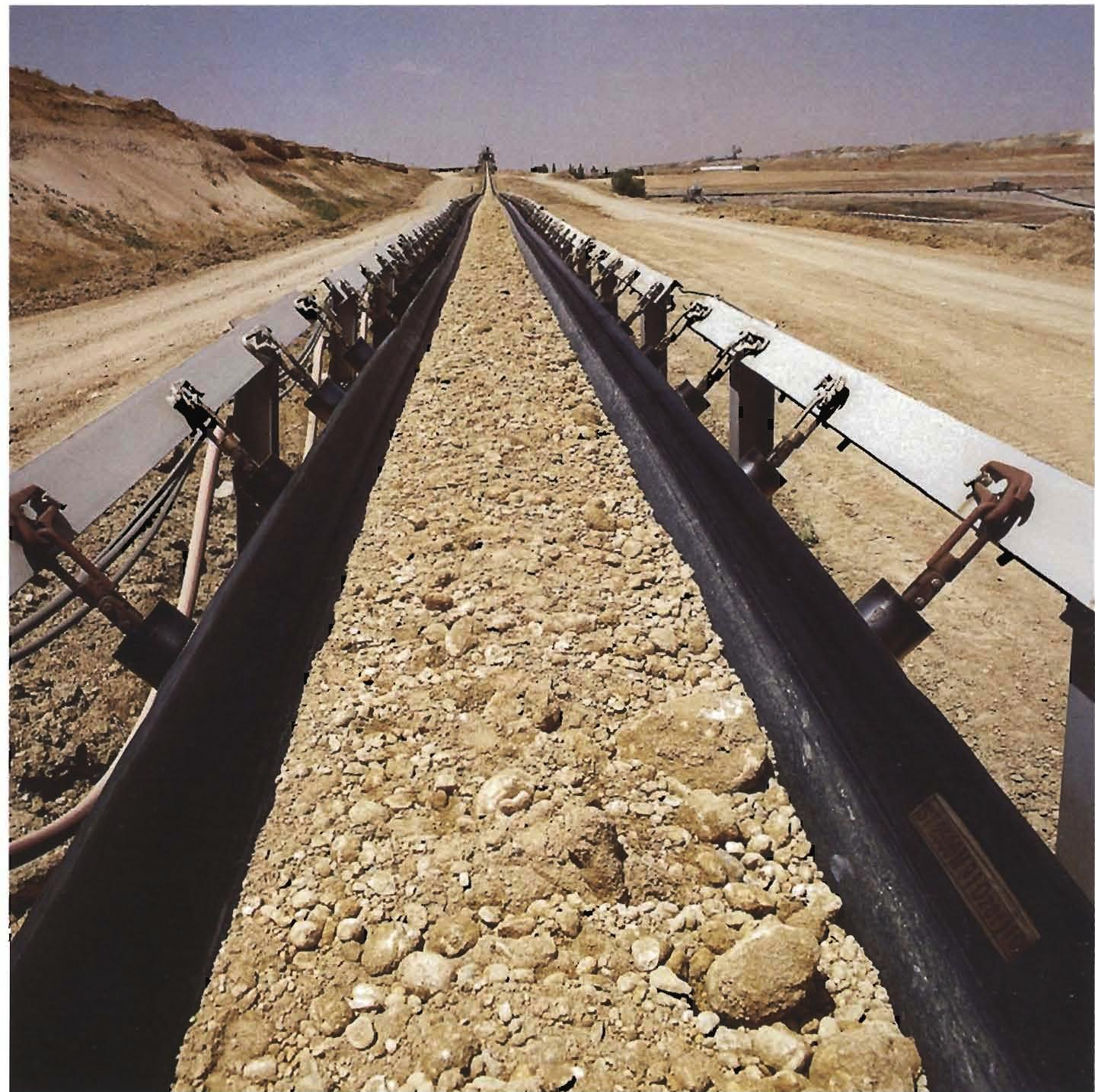
▲ Afşin/Elbistan Lignite Establishments Clay Belt 1800 mm/ST 2500
